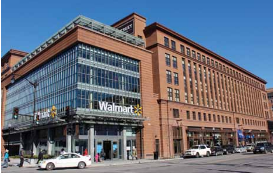
This Walmart on H Street in Washington, D.C., near Union Station features a multi-story design and underground parking.
